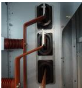
母线室(“I”字型布置) Bus room ("I" layout)
