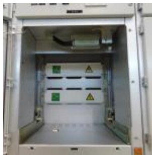
活门关闭 Valve closed
