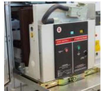
抽出（插入）断路器小车 Pull out (insert) circuit breaker trolley
