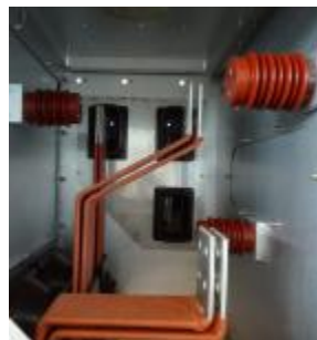
母线室(“品”字型布置) Bus room ("品" layout)
