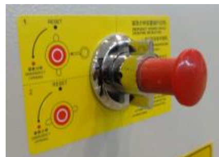
紧急分闸机构 Emergency opening device
