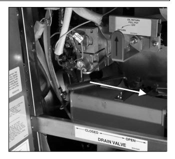
2. Use the steel clean-out rod to clear the drain from **inside** the frypot as necessary.
