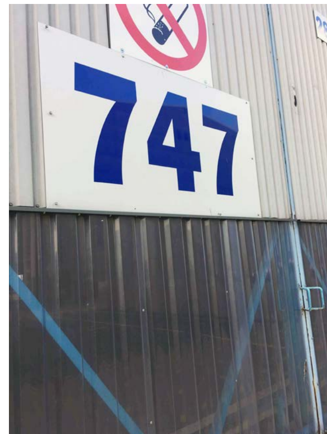
Picture 13. Good example of improved visibility by replacing door lower part with transparent plexiglass
