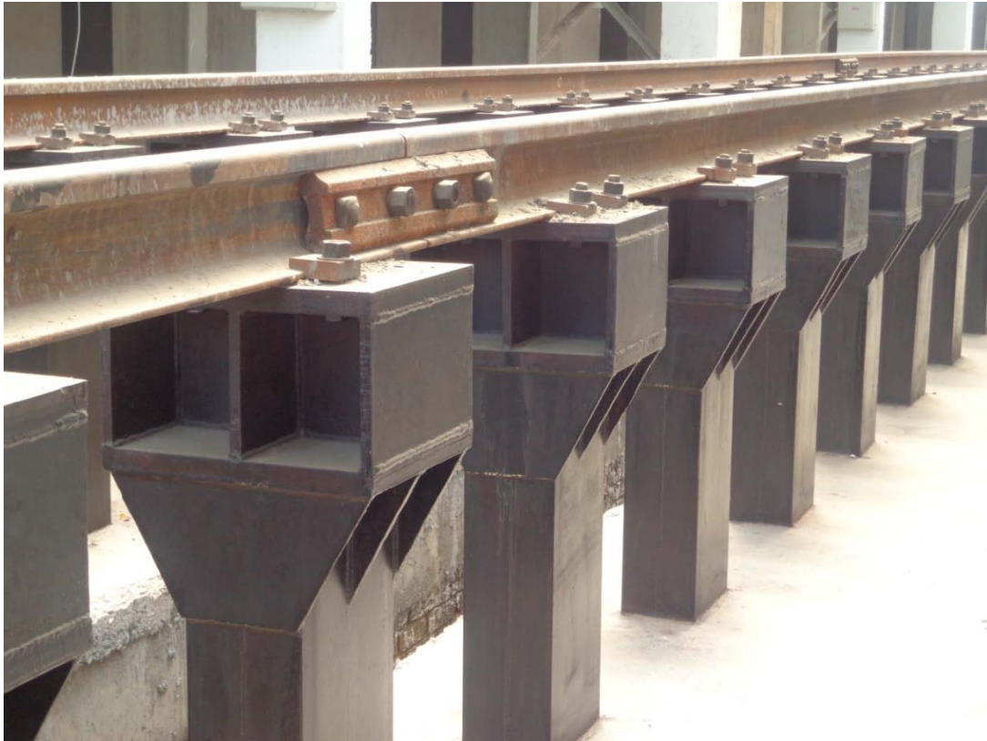
STILT TYPE ARRANGEMENT OF TRACK IN PITLINE
