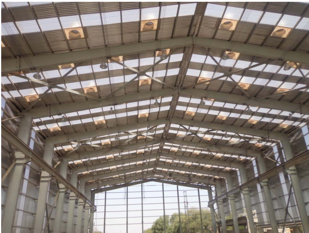
PHOTOGRAPH OF TYPICAL RAFTER ROOF
